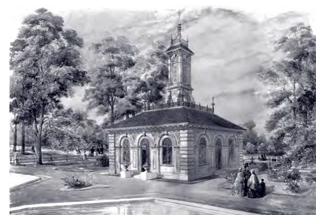
Pump House, Italian Gardens
