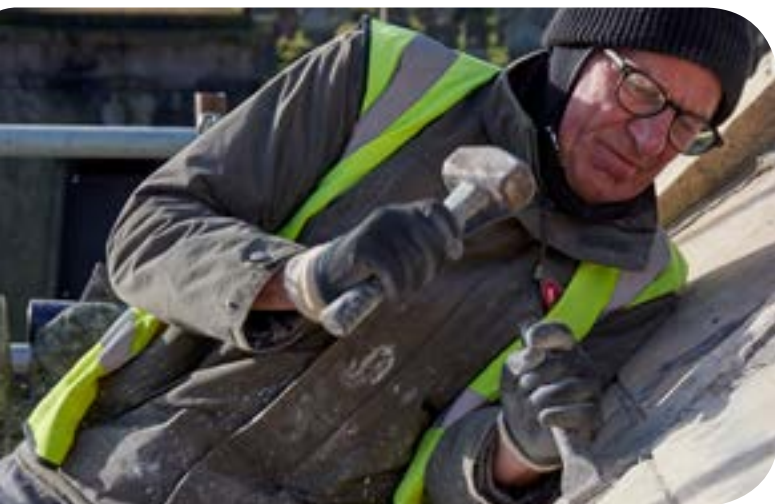
Restoration work at Brompton Cemetery
